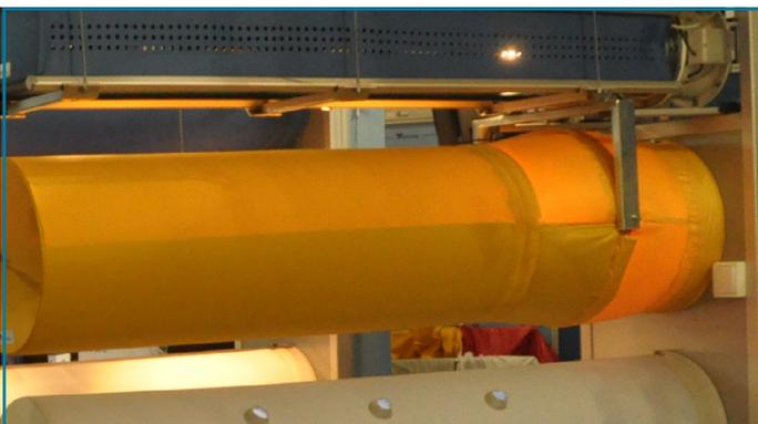
Membrane diffuser - smoke test -video
