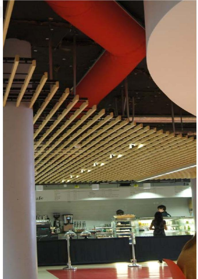
Within this environment Prihoda UK has designed alongside services consultant Mendick Waring, several systems of Textile Diffusers designed to provide Tempered Fresh Air to all of the ground floor library spaces.
