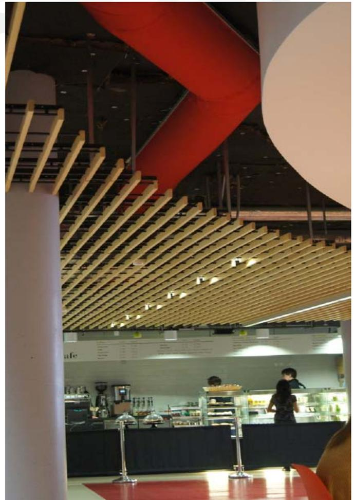
Within this environment Prihoda UK has designed alongside services consultant Mendick Waring, several systems of Textile Diffusers designed to provide Tempered Fresh Air to all of the ground floor library spaces. The Bright Red Textile Diffusers are either exposed against a stark black ceiling or partially exposed between different styles of ceiling furniture – mostly open slats allowing air to filter through into the occupied zone.
